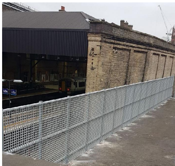
Balconies and Edge Protection
