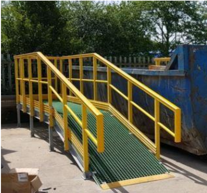
Ramp and Platform
