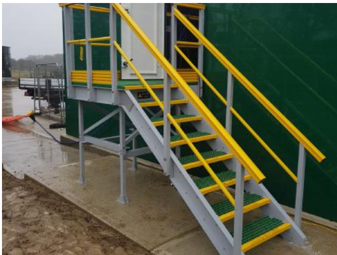
Static Stairs and Platform
